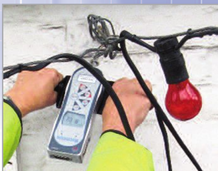
Pull test on anchorage points
